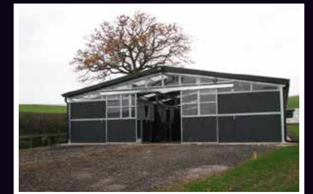
Barn with recycled polyethylene infill
