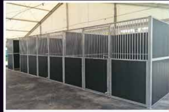
Quarantine Facility, Wellington, Florida
