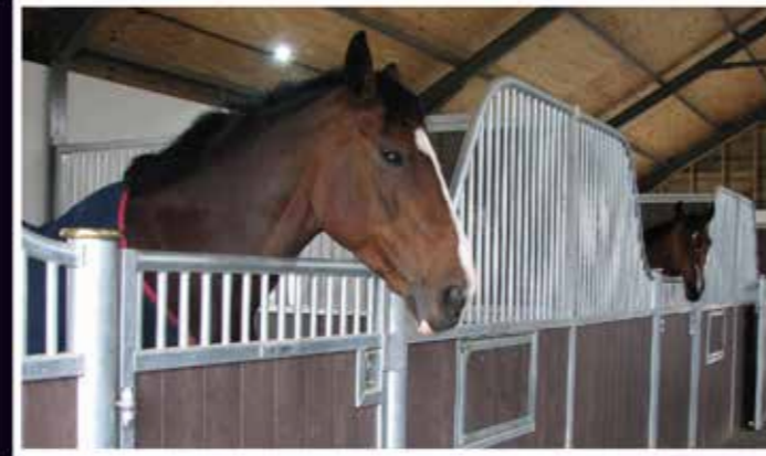
Galvanised steelwork with brown recycled polyethylene infills
