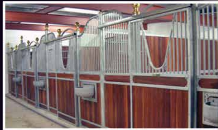
Galvanised steelwork with hardwood infills
