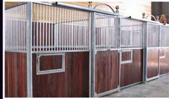
Galvanised steelwork with hardwood infills
