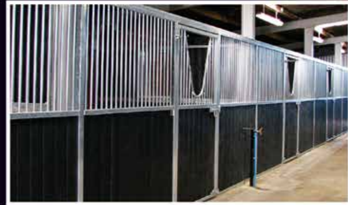
Galvanised steelwork and black recycled polyethylene infills
