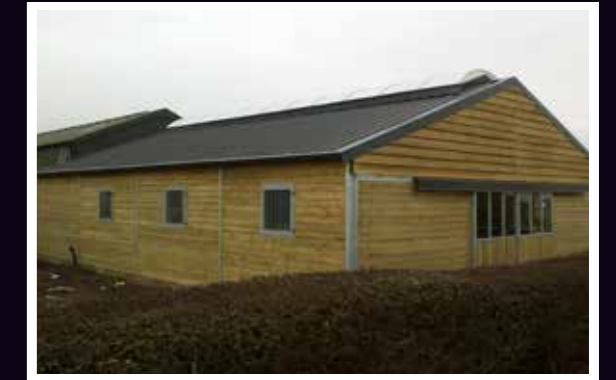
Outside view of barn with ridge light
