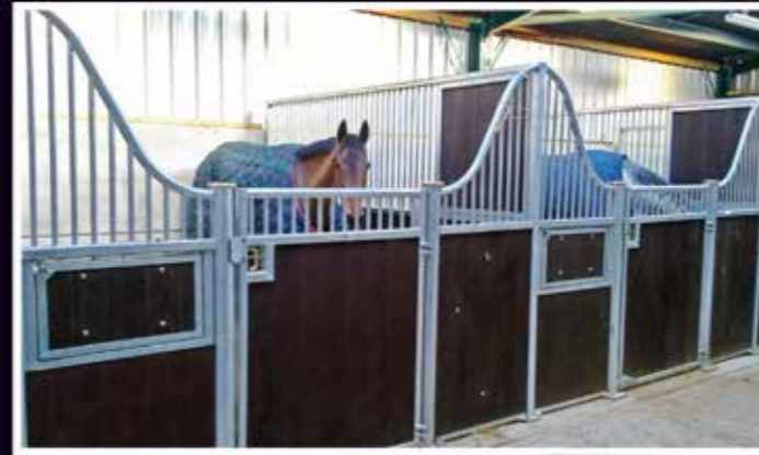
Galvanised steelwork with black recycled polyethylene infills
